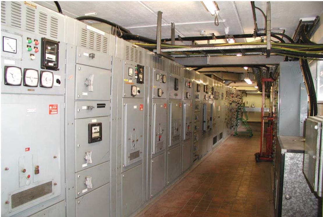
The Ultrasonic test programme identifies issues such as arcing, tracking and corona inside switchgear and will also 'listen' for mechanical issues, such as loose laminations in transformer cores.
