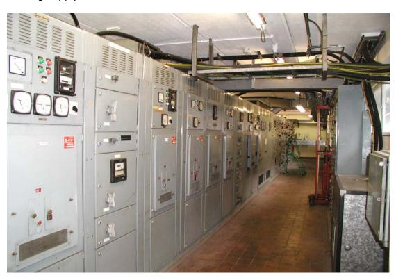
The Ultrasonic test programme identifies issues such as arcing, tracking and corona inside switchgear and will also 'listen' for mechanical issues, such as loose laminations in transformer cores.
